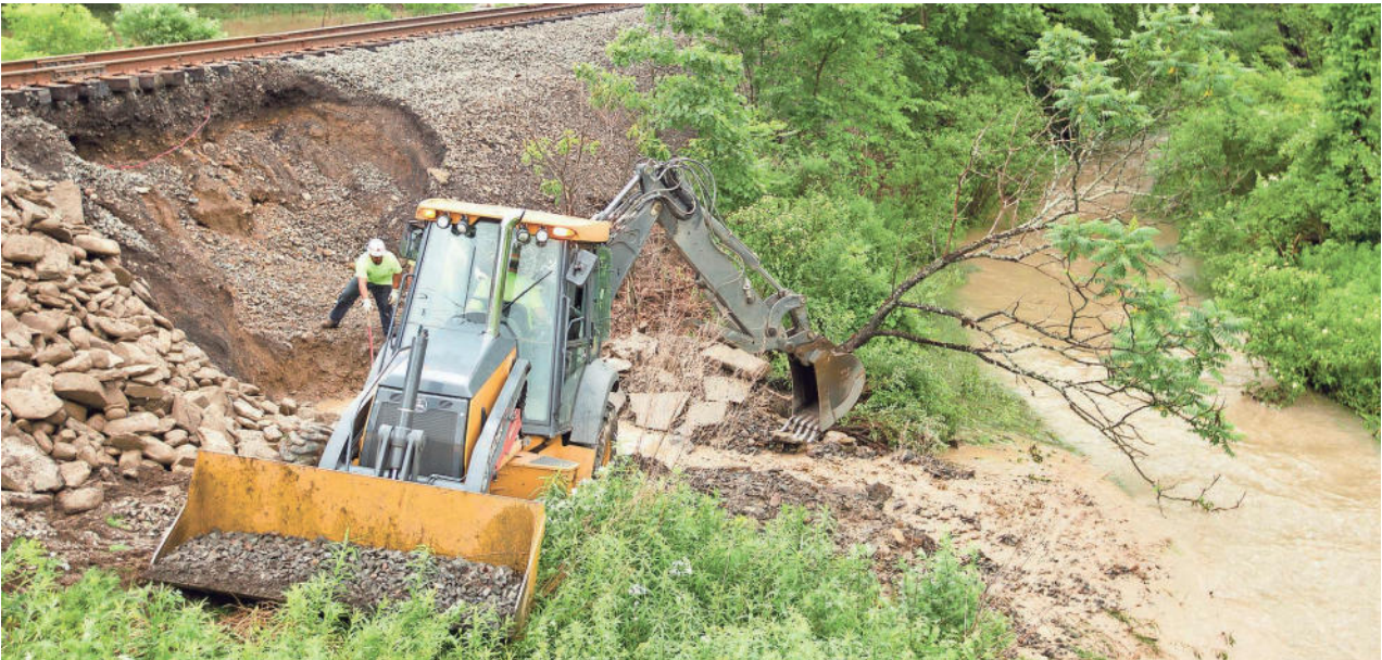
A crew with Norfolk Southern railroad works Tuesday to clear a plugged culvert under the track that crosses Station Road in the Town of Danby.
