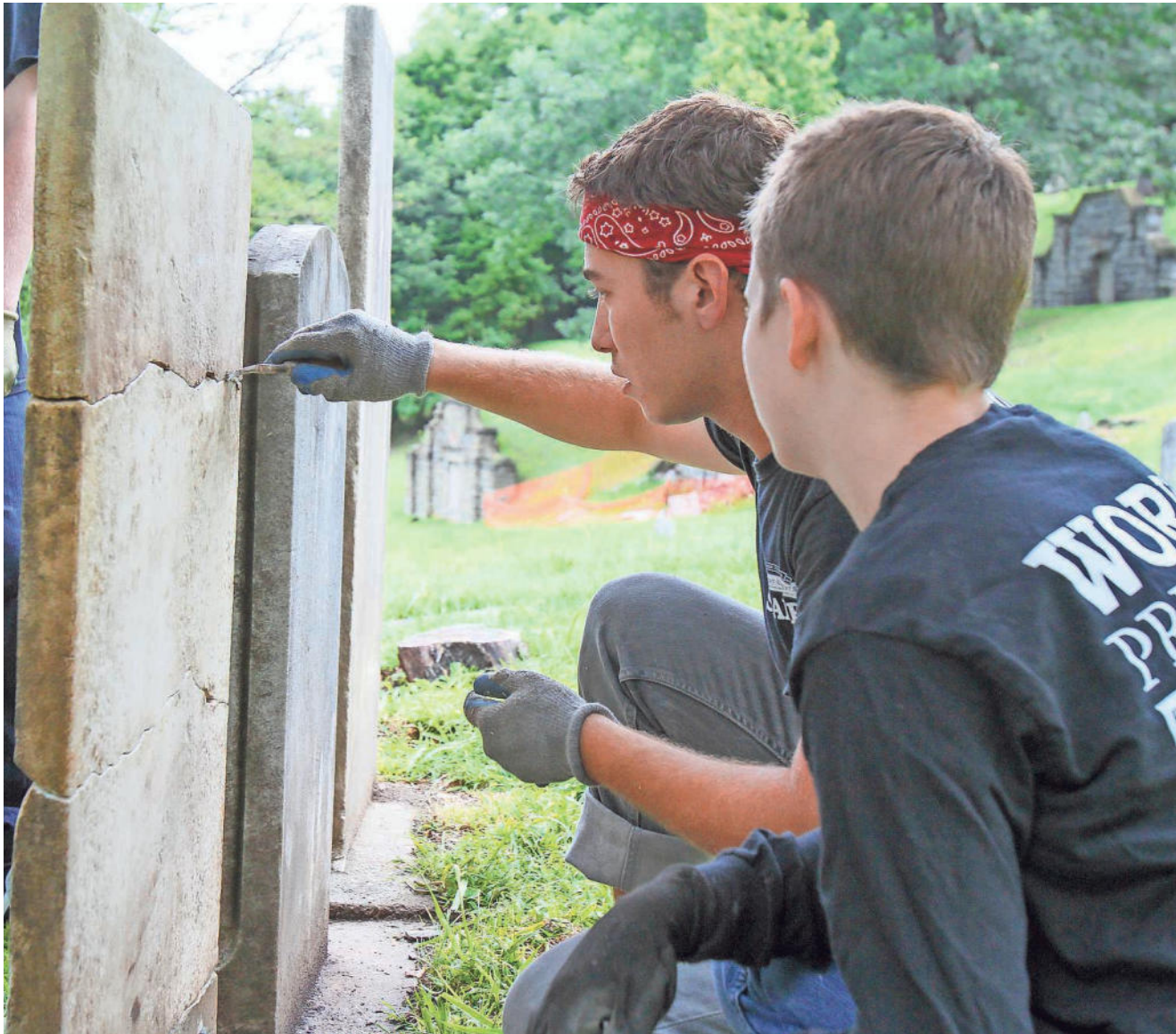
Randy Ruth, rear, shows Alexis LaPage, 16, how to repair a headstone using mortar.
